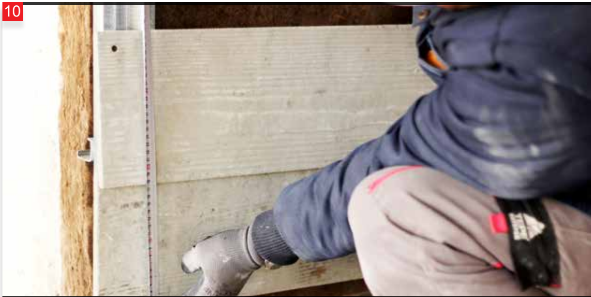
Measurements are taken for the subsequent panels.
