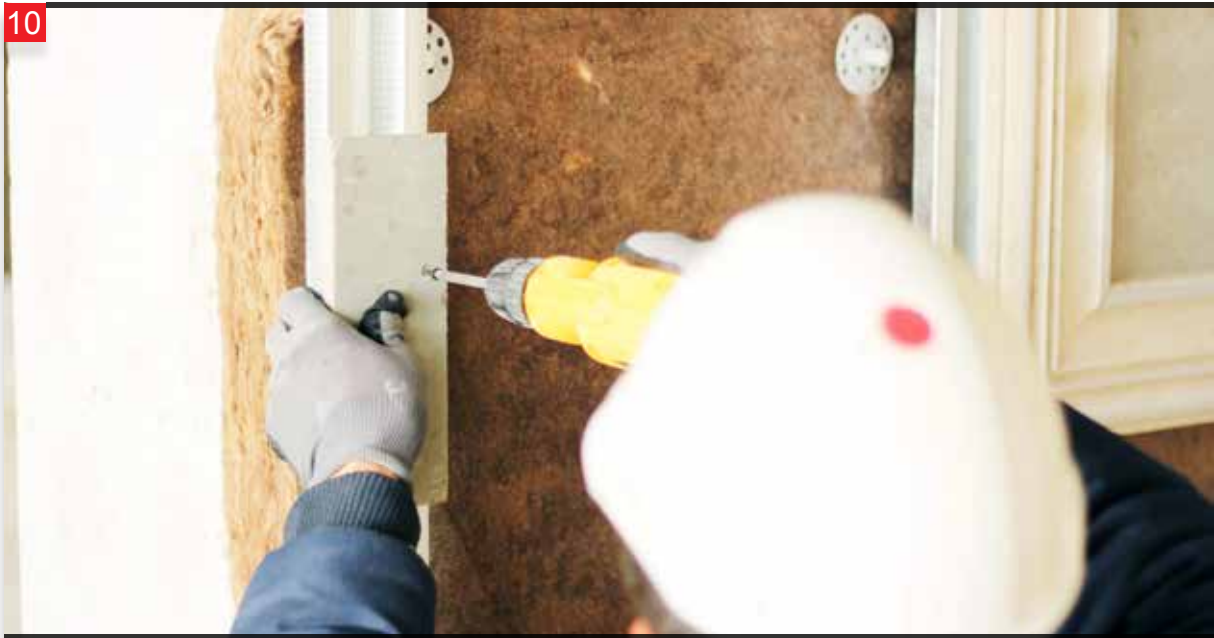
Balancing strips are placed on the middle sections of the area where the next panel will come.
