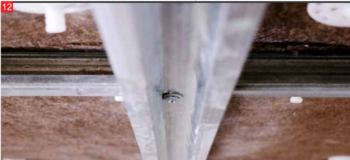
The M profiles that are used should be galvanized 20x80x3000 mm size and 0.50-0.55 mm thick. (The M profile dimensions and thickness may vary according to the static calculation).
