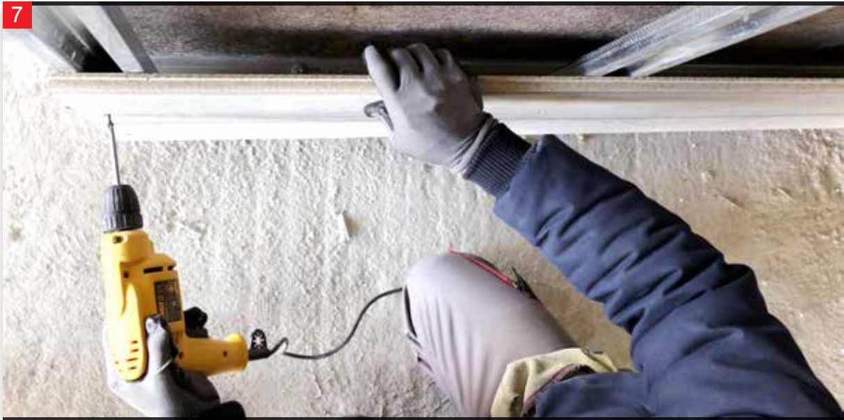
The aligned panels are screwed onto the M profile with drywall screws.
