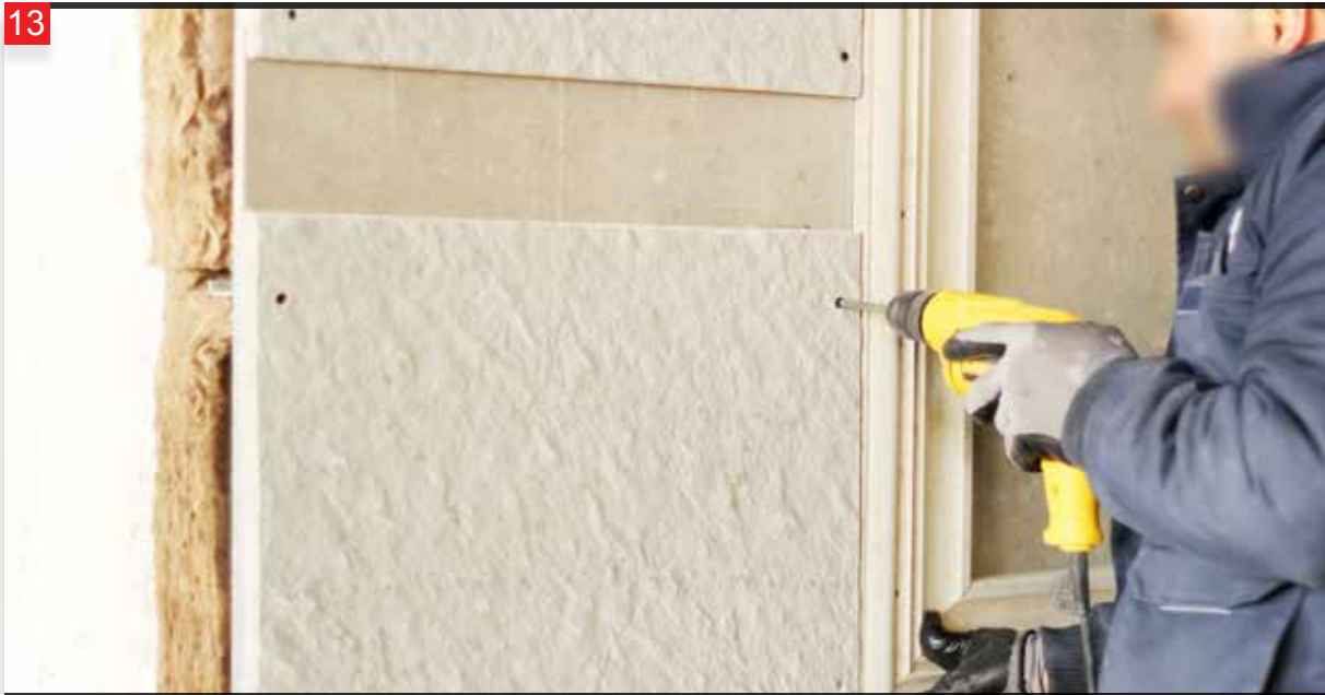
The screws need to be 2.5 cm in from the top and bottom edge.
