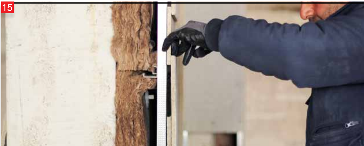
Carbon coated anti rust drywall screws should be used and driven in vertically.
