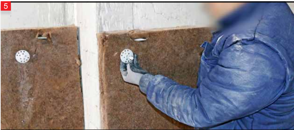
The desired thickness of insulation material is applied on the fixed L consoles.
