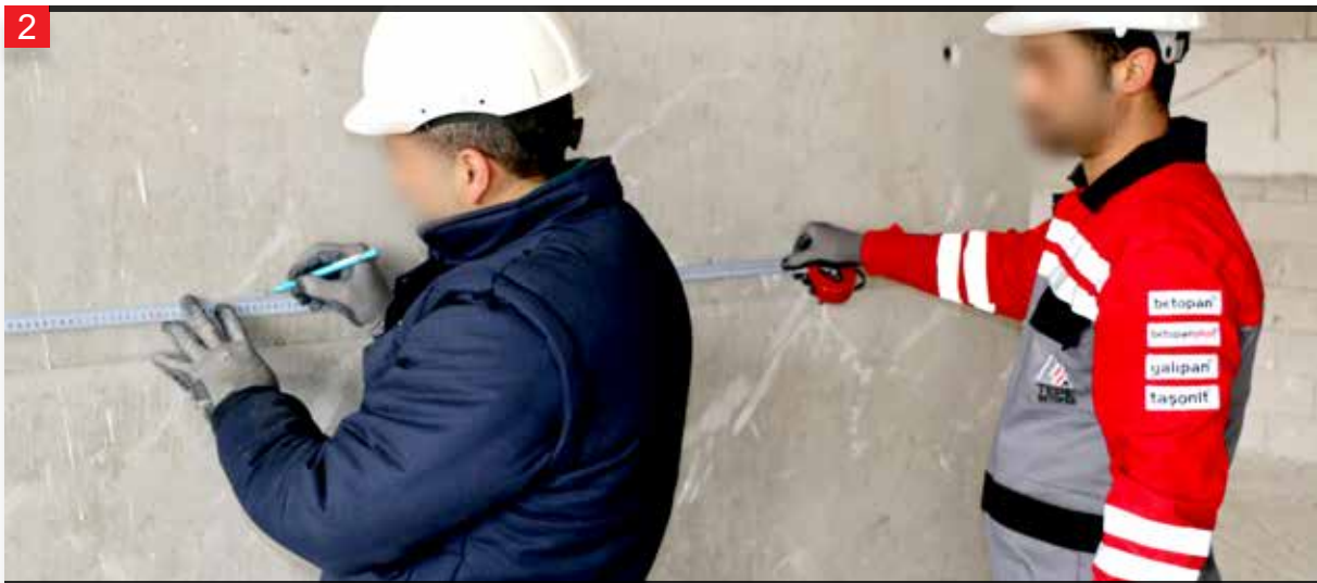
The position of the L consoles are determined and marked at 1 meter intervals. (May vary according to static calculation)
