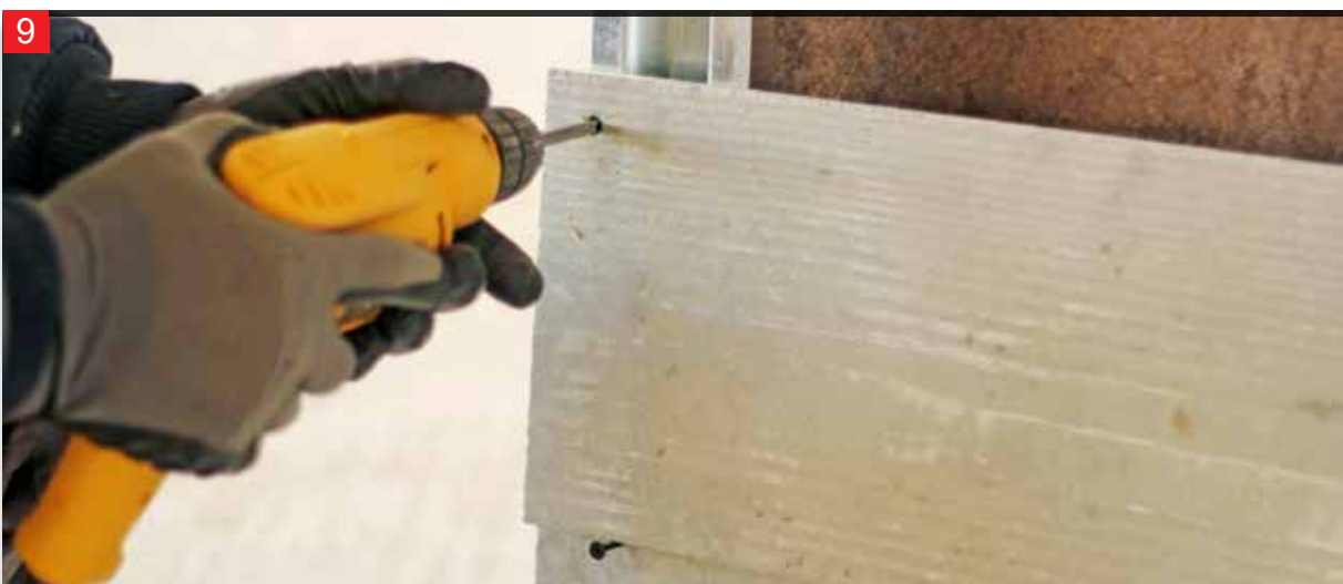
Carbon coated anti rust drywall screws should be used and driven in vertically.
