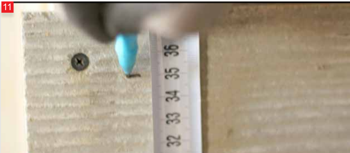
2,5 cm distance from the top is left for the overlapping surface.
