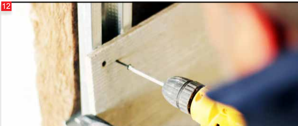
Screws are driven into the measured points as a guide to the overlapping panels.
